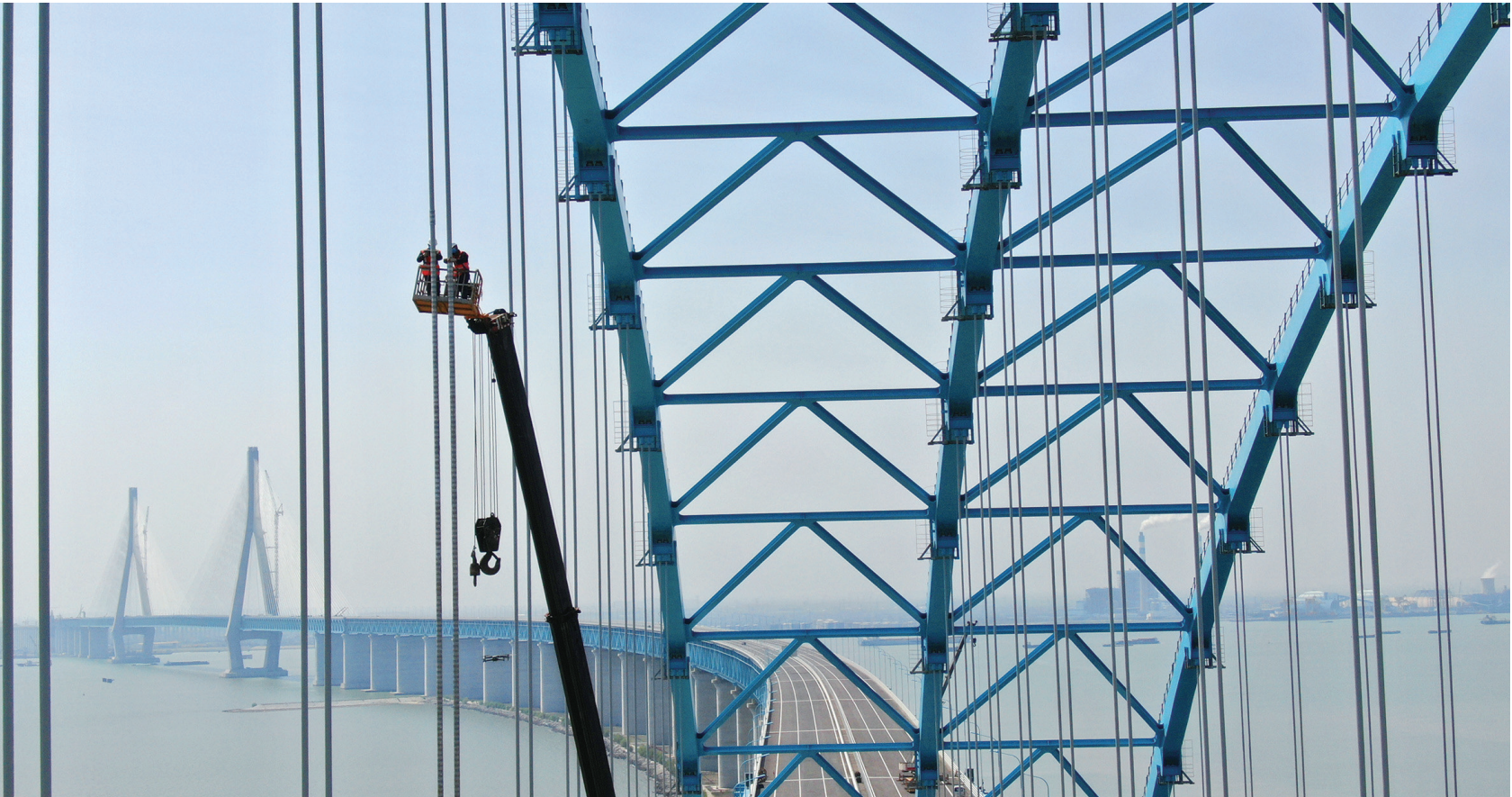
On 2 April, workers were installing pressure ring sensors of the cable of Hutong Yangtze River bridge Tiansheng harbour channel bridge up in the air, and adjusting the cable according to loading conditions of the bridge cable obtained from the sensors. Cable adjustment work is estimated to be completed by 10 April. Photo by Xu Congjun
