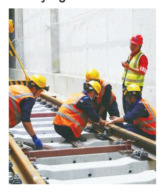
On 26 August, as a group of 25meter-long rails were lifted to the designated places from rail base, Nantong rail transit line No.1 rail laying was started.
