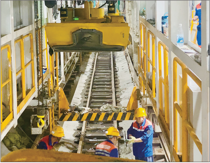
Workers were installing the rail. Photo by Peng Junjun
